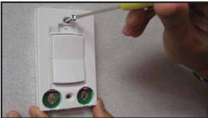
Figure 2. Mounting Wireless Wall Switch
